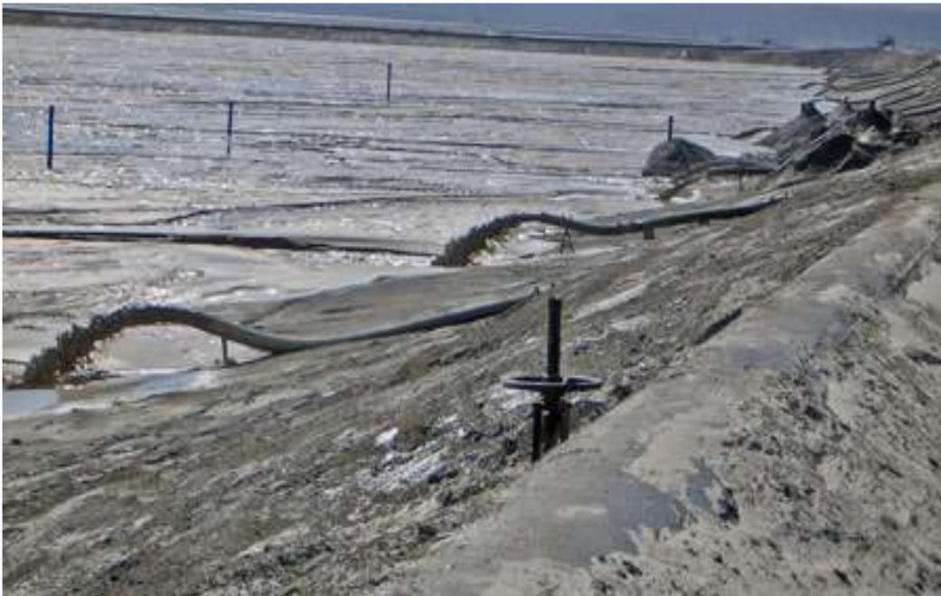
**Figure 1.2:** Discharge of slurry into Tailing Storage Facility
