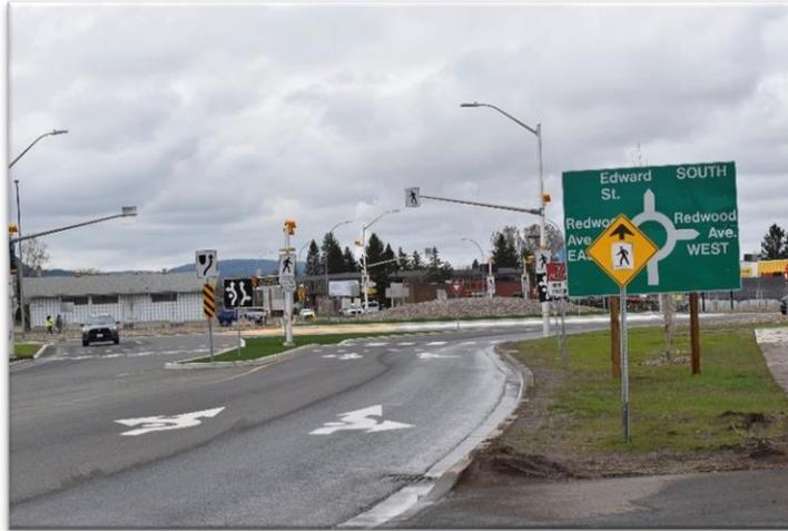
**Figure 14: The Roundabout in Thunder Bay with the “Pedestrian Crosswalk Ahead” (WC-2) sign**
