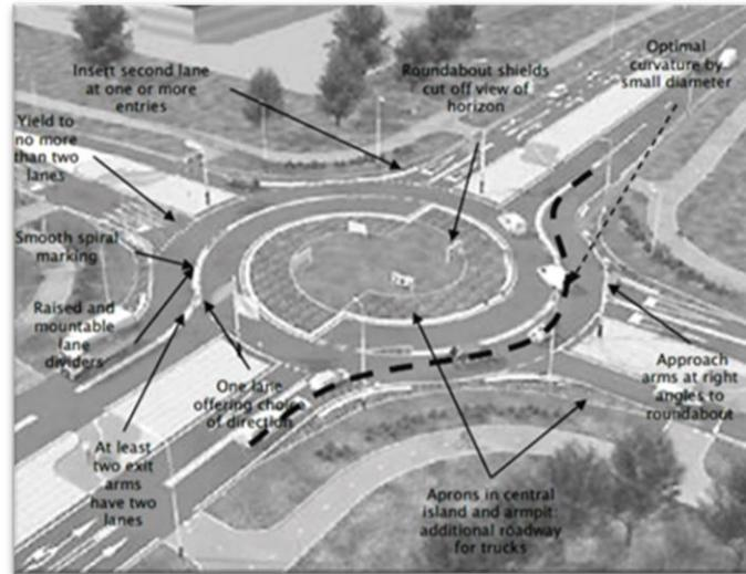
**Figure 4: A Turbo Roundabout [11]**
