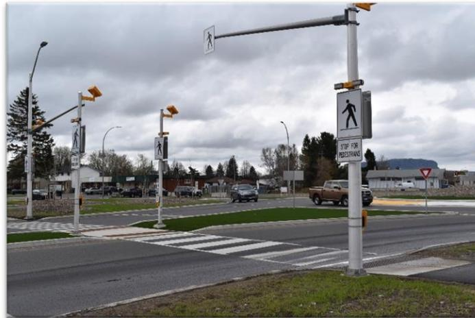
**Figure 13: The Roundabout in Thunder Bay with the “Pedestrian Crosswalk” sign**
