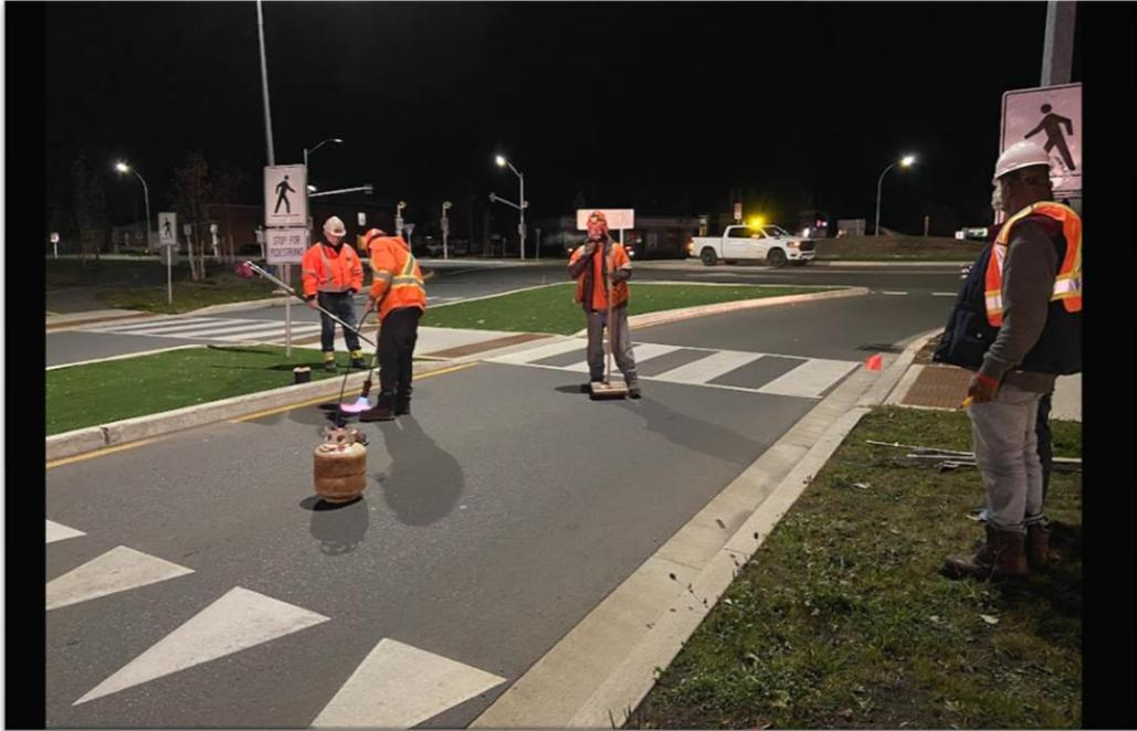
**Figure A13: Cleaning the surface with a broom, followed by drying the surface with a blow torch before installing the strips at about 5 am local time on Thursday, October 27, 2022**
