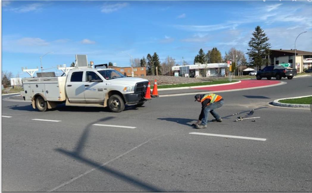
**Figure 26: Strips being removed from the road**
