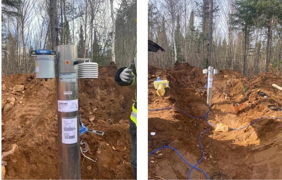
Figure 5. A Lakewood Systems remote data logger housing (RDH) was installed in a trench at roadside and sensor wiring routed to a datalogger inside. A rain gauge and air temperature radiation shield assembly were mounted on the left and right sides, respectively, of the RDH.
