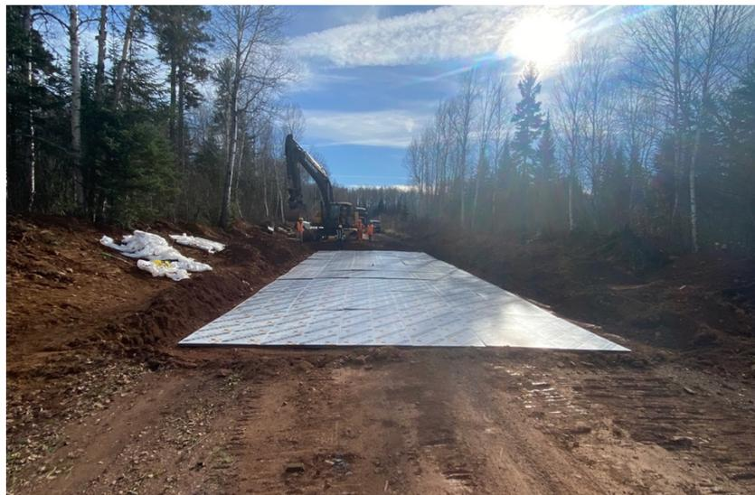
Figure 3. Southbound view of test section 1 prior to covering the insulating layer.
