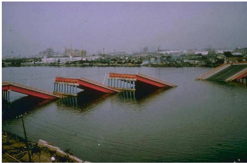
Figure 1.4 Showa Bridge after Niigata earthquake [8]
