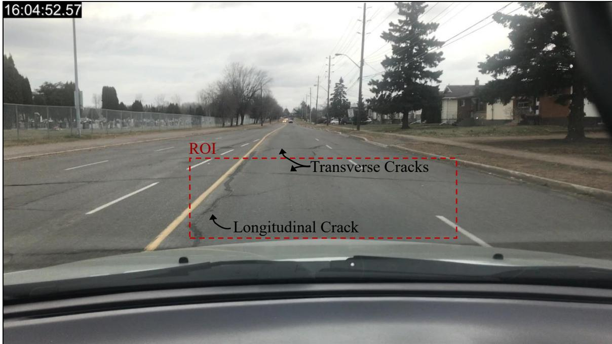
**Figure 62. Cracks in the road that could cover multiple extracted frames**
