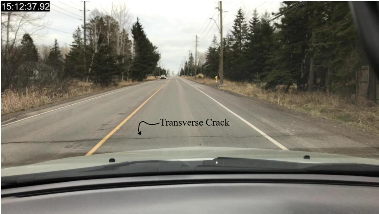
**Figure 59. A difficult to detect transverse crack in the road**
