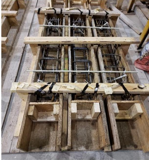
**Figure 3.2.** Formwork and reinforcement of cast columns
