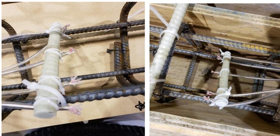
**Figure 3.5.** Thermocouple installation in a general column's formwork
