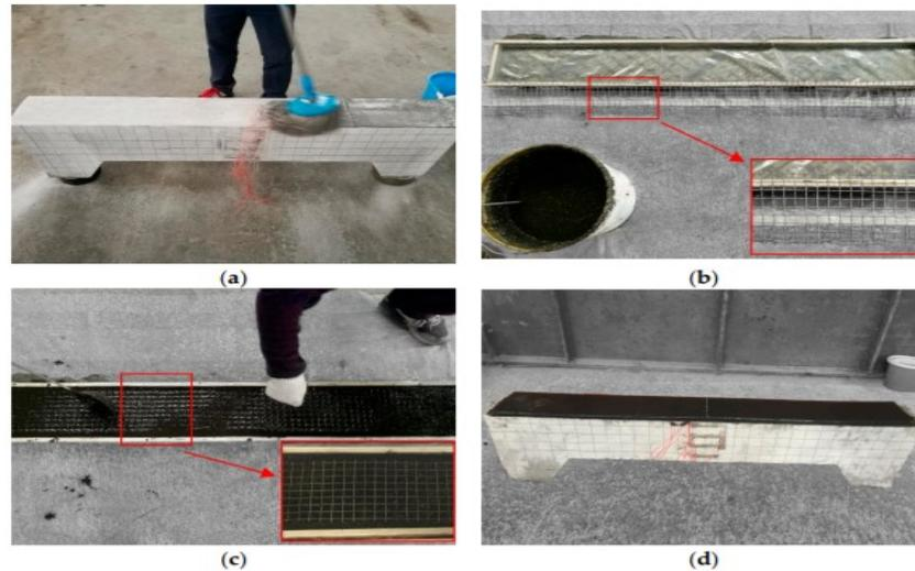
**Figure 2.4.** Strengthening process: (a) clean and wet surface; (b) installing formwork; (c) installing steel mesh; (d) cast resin concrete (Adapted from Li *et al.*, 2018)
