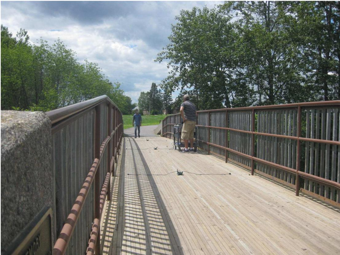
Figure 4.12: Pedestrian bridge on the campus of Lakehead University instrumented with wireless sensors
