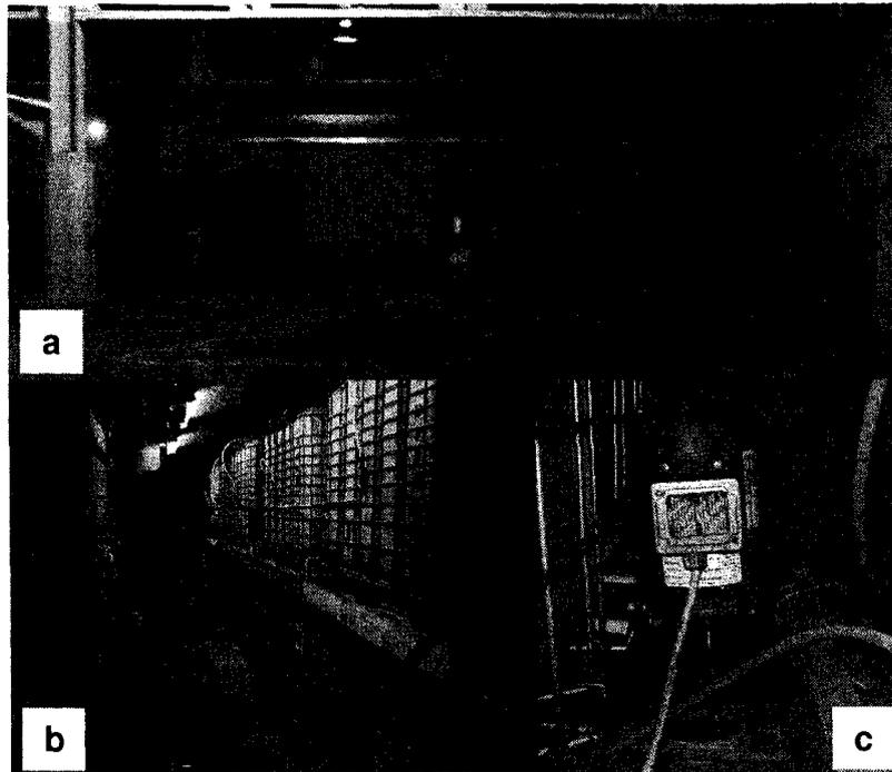
Figure 7 - Effluent storage for the flow-through experiments: a – cold room (outside) on 3<sup>rd</sup> floor of AbitibiBowater newsmill. b - cold room (inside) and 1050L storage tanks. c - agitator motor used for stirring and dechlorination
