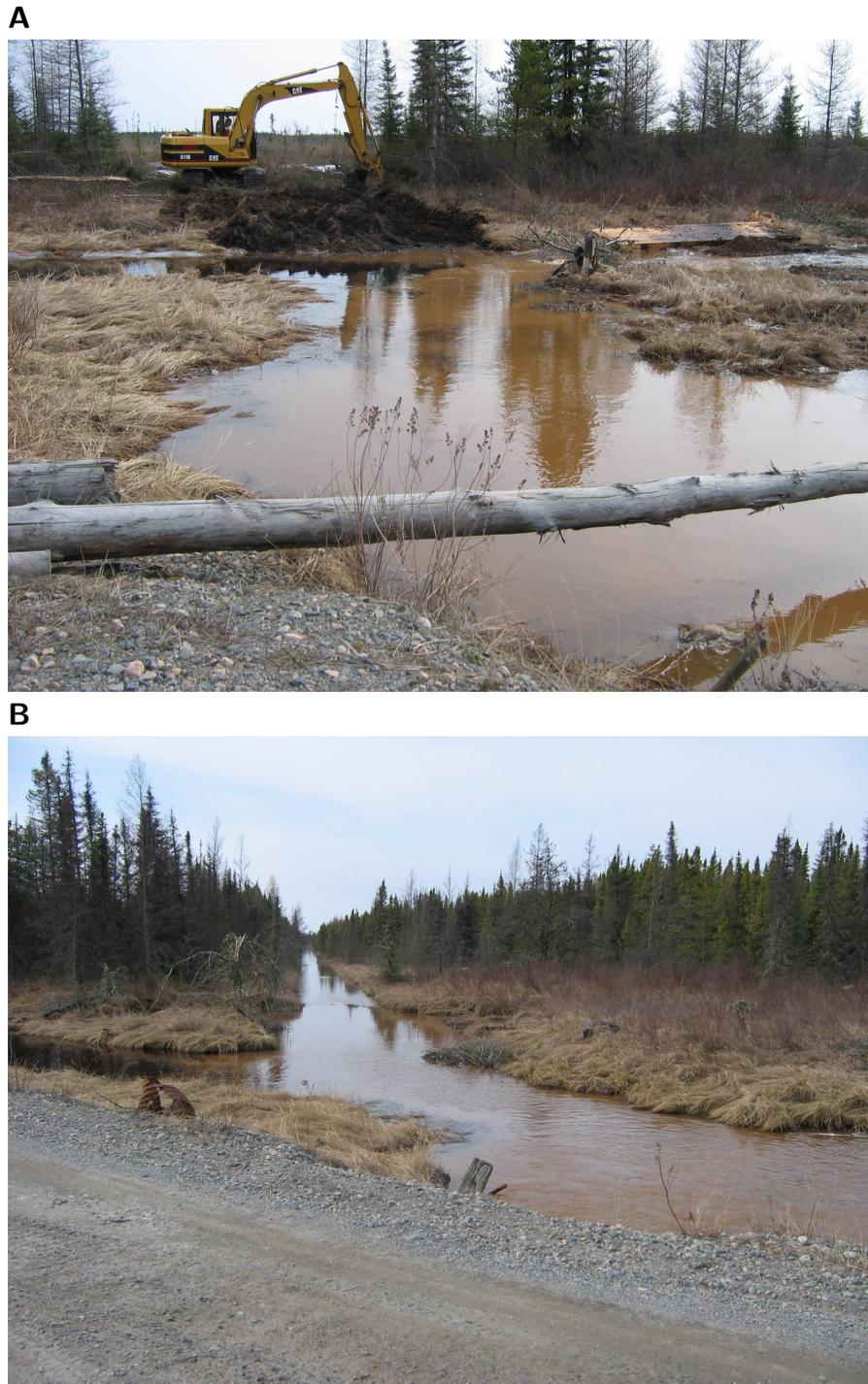
Figure 2.15: Observational evidence of solids discharged during active wet peat mining. Photo **A** was observed from the road atop the culvert location, looking upfield towards the experimental wet mining study site. Photo **B** was observed from the same location, looking downstream towards the receiving water ecosystem that consisted of pre-existing drainage ditches (circa. 1940's). See Fig. 2.1 for schematic representation.
