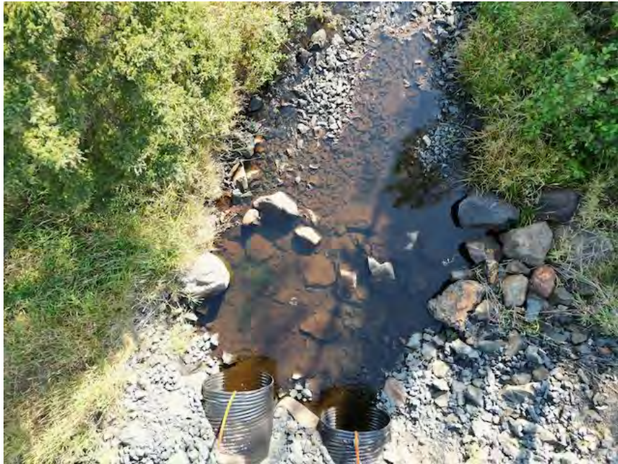
Figure 3.10 Hazelwood Drive Study Site
