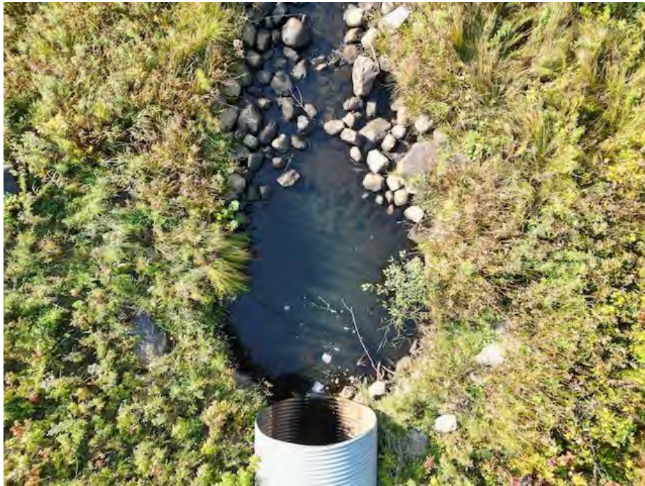
Figure 3.14 Road 527 Study Site
