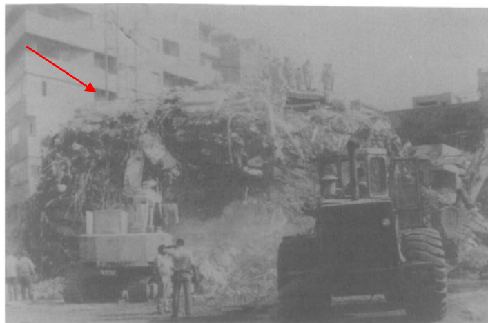
Figure 2.4. The complete collapse of a 14-storey reinforced concrete residential building in Cairo adapted from (Badawi and Mourad, 1994)
