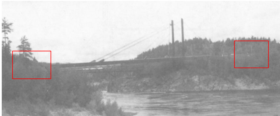
Figure 2.10. Overview of the constructed 1992, double-leg steel cable-stayed Shipshaw bridge of 183 m in length, adopted from (Filiatrault et al., 1993)
