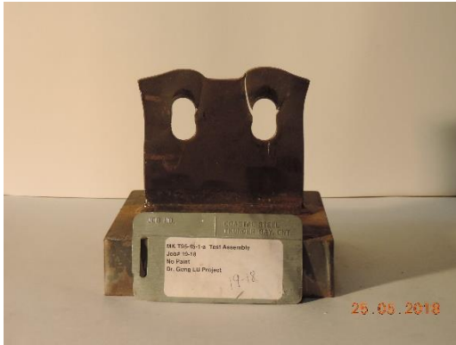
T95-45-1-a: bearing tear-out
