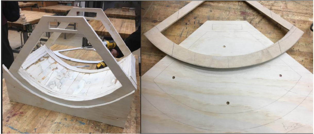
Figure 3.8: The carpentry stages in the construction of wooden PV frame.
