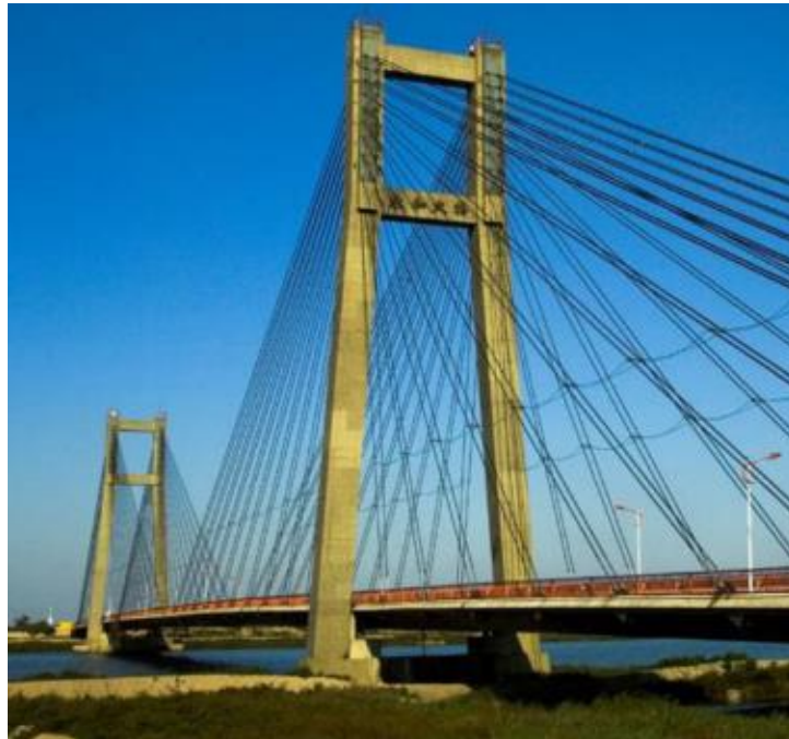
Figure 5.1: General view of the investigated bridge [73].
