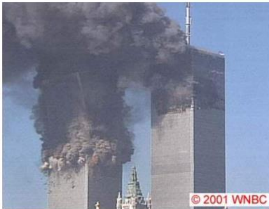
Figure 2.5: Collapse of WTC tower 2 after the 9/11 terrorist attack [21].
