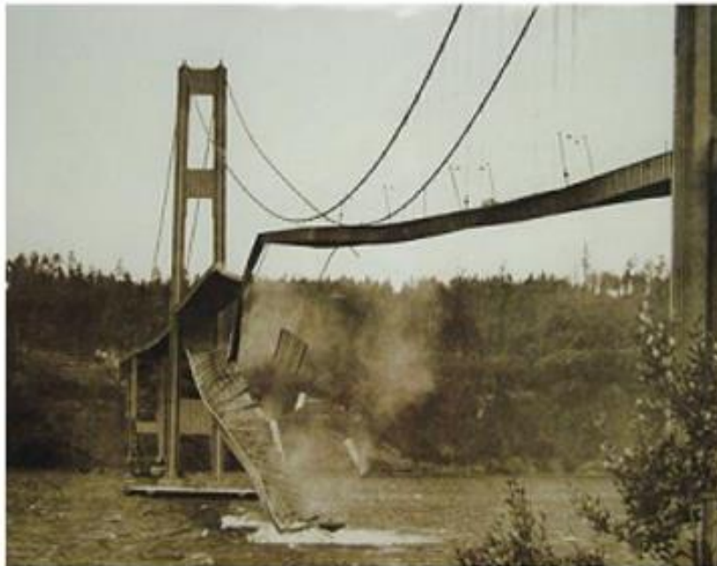
Figure 2.2: After the collapse of Tacoma Narrows bridge [19].
