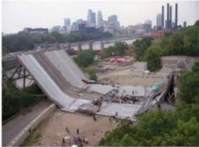
Figure 2.4: After the collapse of 35W bridge [21].
