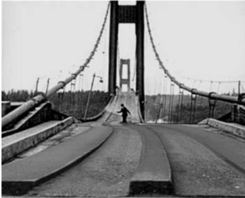
Figure 2.1: The start of the collapse of Tacoma Narrows bridge [19].
